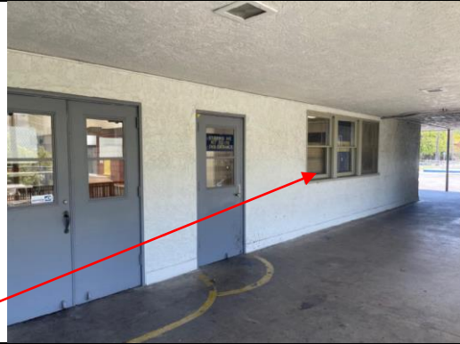
Photo of lead-based tan wood window casing on the exterior of the Cafeteria.
