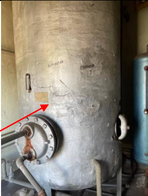
Photo of asbestos-containing white boiler tank insulation in Weight Room/Museum Building.
