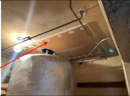
Photo of asbestos-containing white drywall and joint compound (patch) in Cafeteria Building.
