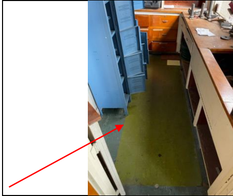
Photo of asbestos-containing blue/green 9"x9" floor tile in Weight Room/Museum Building – Equipment Room.
