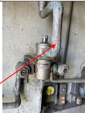
Photo of lead-containing silver metal pipe in Mechanical Room.
