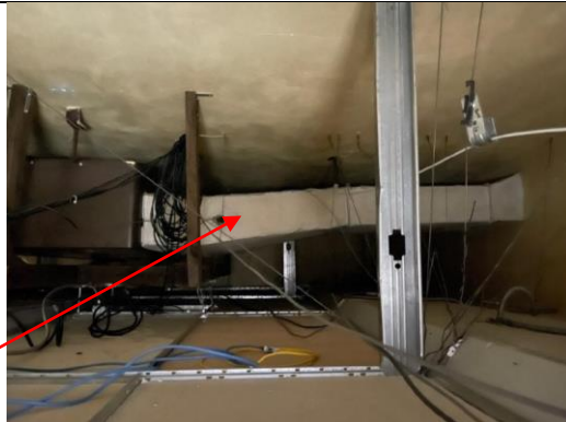
Photo of asbestos-containing gray corrugated ducting in Weight Room/Museum Building.
