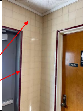
Photo of lead-based beige and white ceramic walls in Weight Room/Museum Building – Main Corridor.
