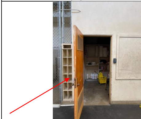
Photo of lead-containing tan wood cubbies in Weight Room.
